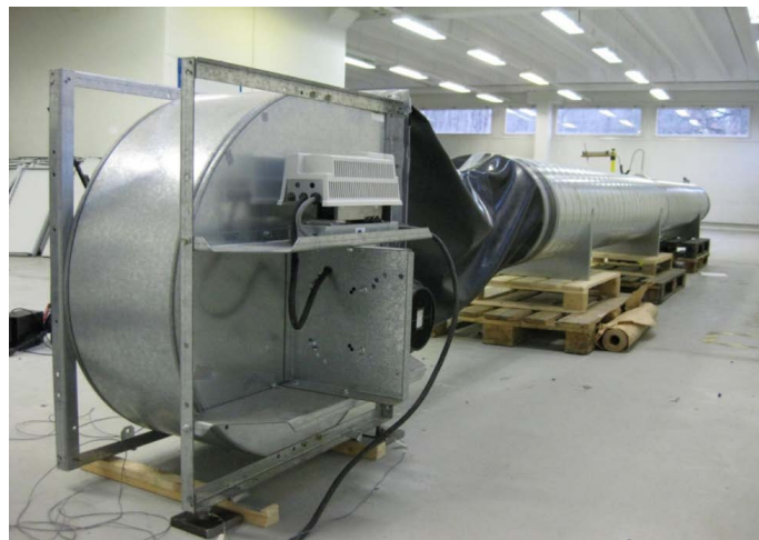
Figure 6: Photograph of the test set up.
